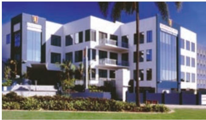
R&D Centre and Head Office, Brisbane
